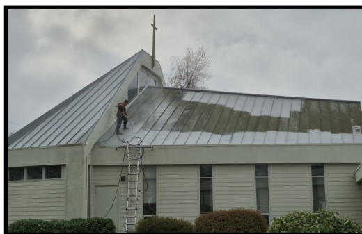
Sanctuary metal roof cleaned.
