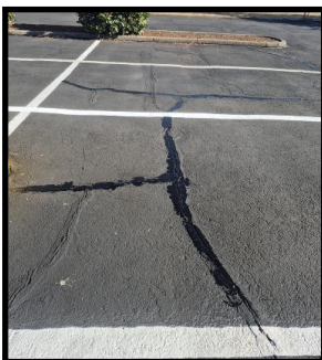
Parking lot before and after new crack sealant and striping.
