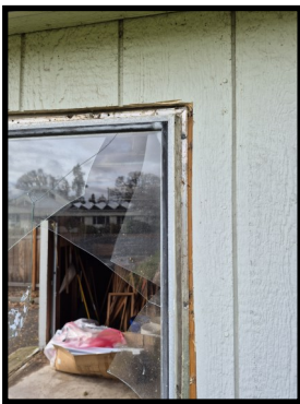
Repair shed window and siding from vandalism damage.
